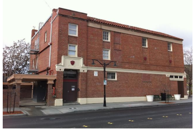
109 J Street Façade & Entrance
